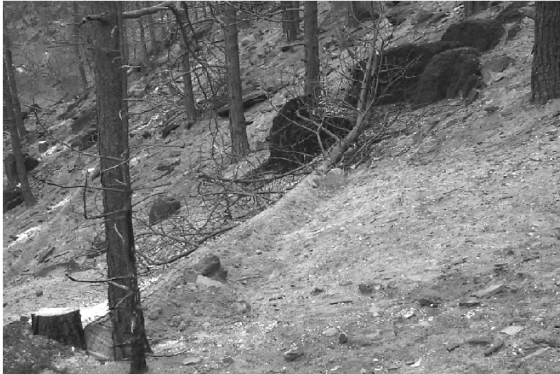
Figure 3. A contour felled log installed immediately after the Bobcat wildfire in the Colorado Front Range. The trench upslope of the log is created by excavating the soil and packing it against the log to prevent underflow (from Wagenbrenner et al. 2006).
