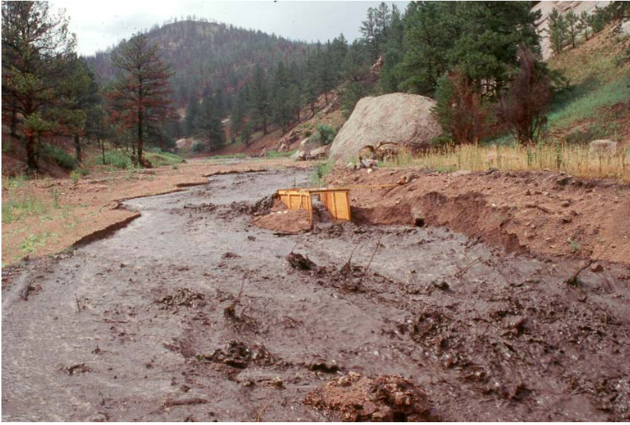
Figure 5. After a high-severity fire runoff can bypass or greatly exceed the capacity of a flume installed to measure discharge. Picture taken after the 1996 Buffalo Creek fire by John Moody, USGS.
