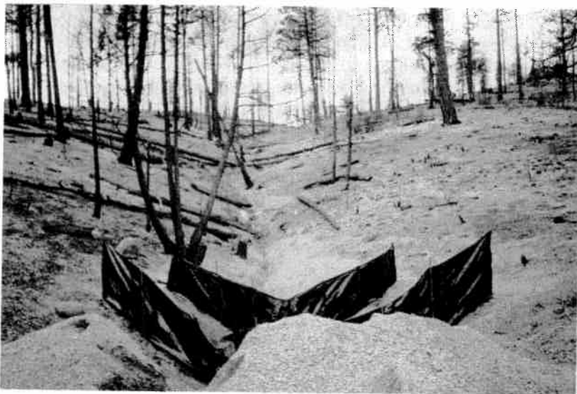
Fig. 2 Photo from summer 2003 showing a pair of sediment fences, the piles of sediment excavated from the fences, and the relatively bare hillslopes one year after the June 2002 Hayman Fire.
