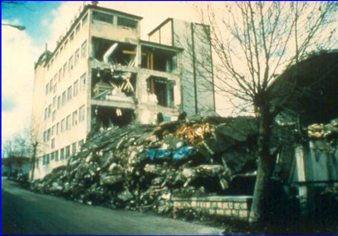
Factory collapse, Italy 1980 (M = 6.9)
