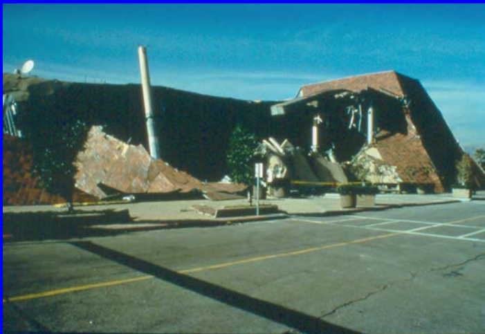
Factory collapse, Italy 1980 (M = 6.9)
