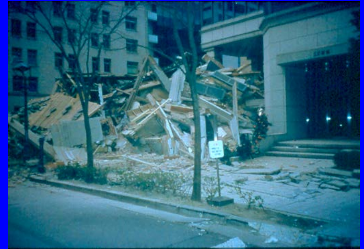
Total collapse of Buddhist temple, while modern quake resistant buildings are left standing. Kobe, Japan 1995 (M = 6.9)
