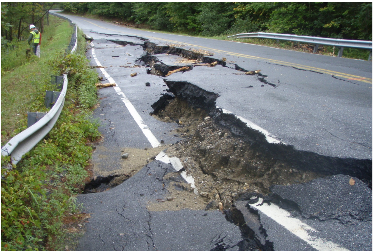
Figure 11. Slip scarps in roadway at Slide 1 due to rotational slumping. Slumping caused by erosion of toe, excess pore pressure, low strength soils and excess loading from precipitation.
