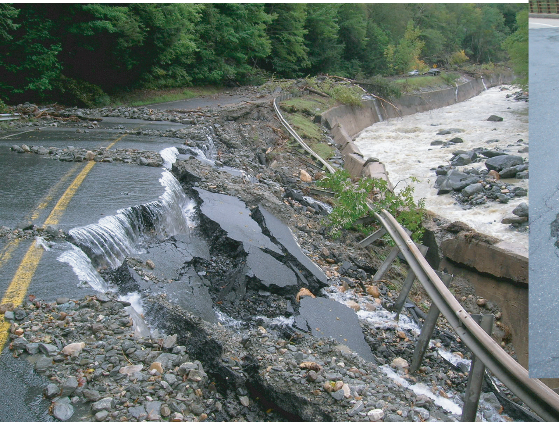
Scouring exposed footings of retaining wall and overflow on road surface due to clogged cross culverts caused erosion of roadway and eventual toppling of retaining wall.
