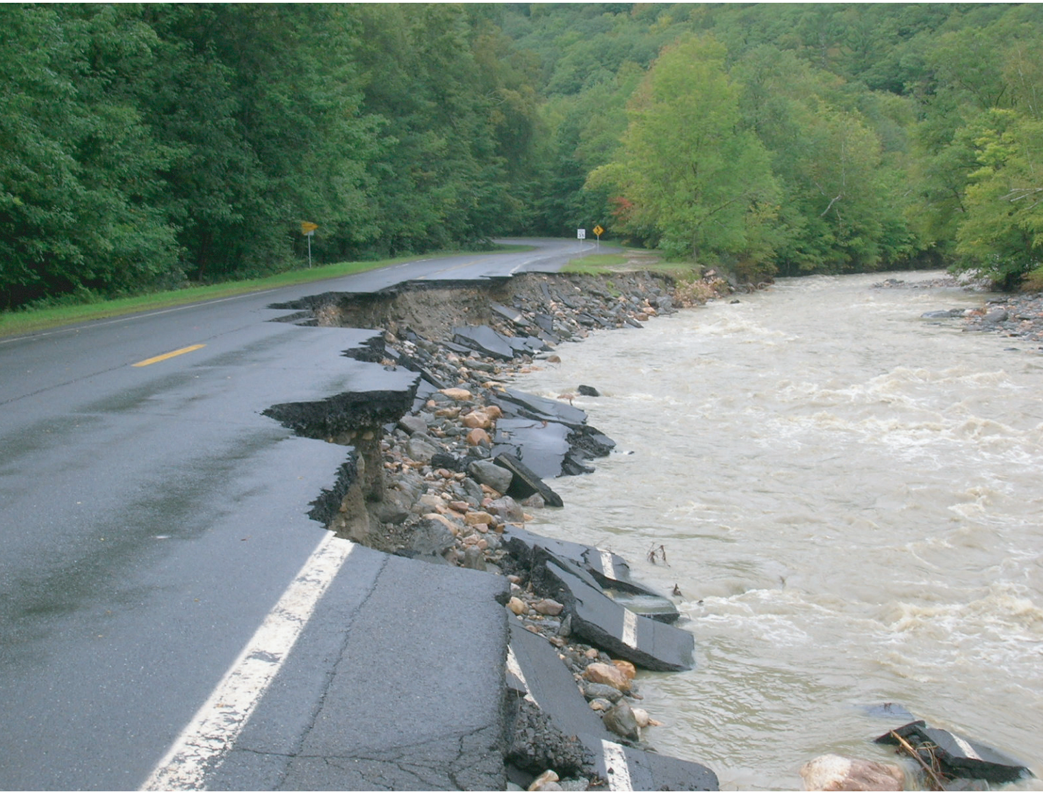
Fluvial erosion damage along Route 2. This repair is estimated at $3 million.
