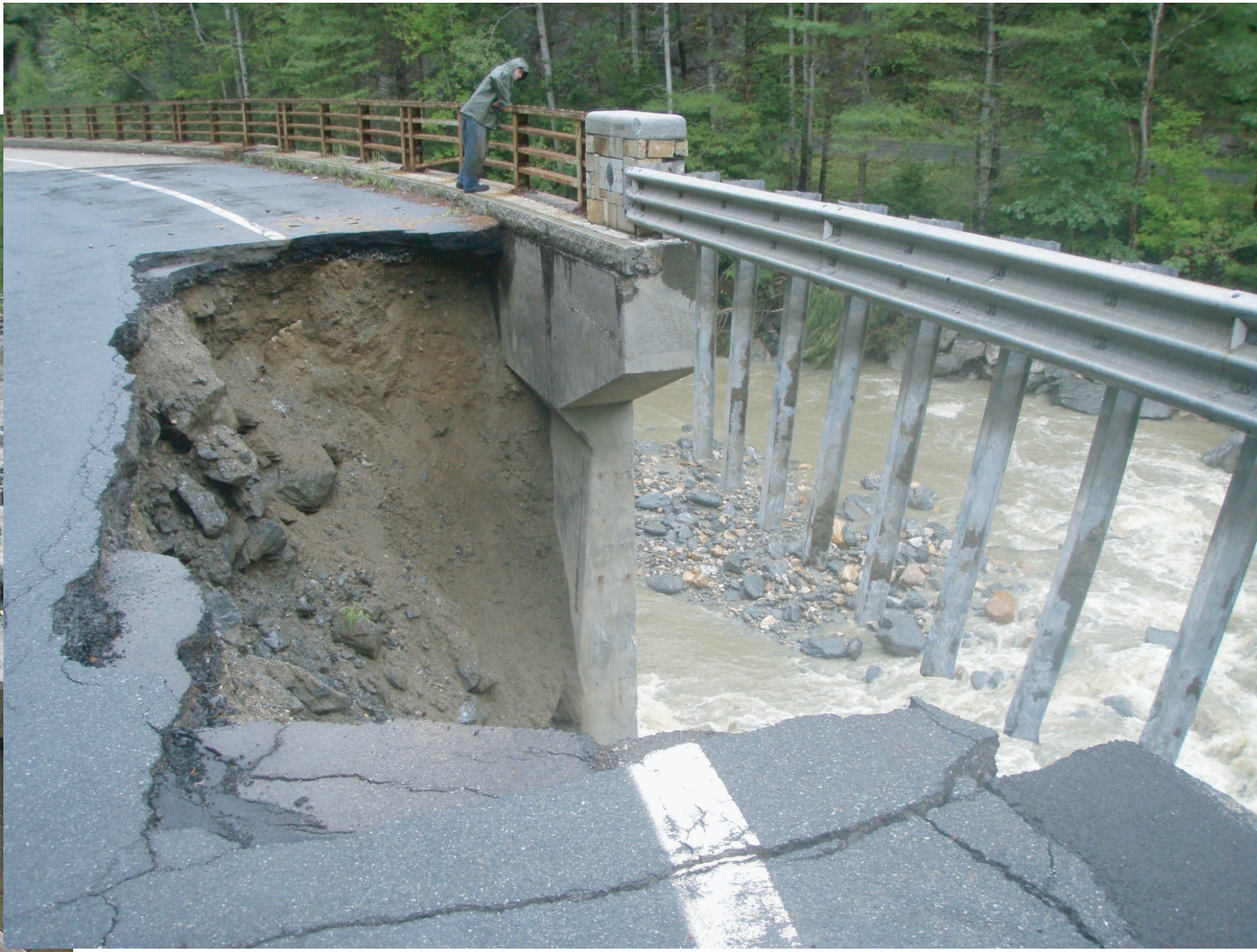
Bridge over Cold River in Savoy at intersection with Black Brook. This bridge was not overtopped. Violent eddies at downgradient end of abutment eroded the backfill and undercut road surface causing collapse. This phenomenon was observed at many bridge crossings.
