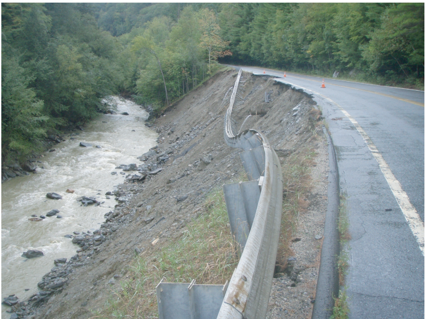
Erosion damage to unreinforced embankment on Route 2 along the Cold River.
