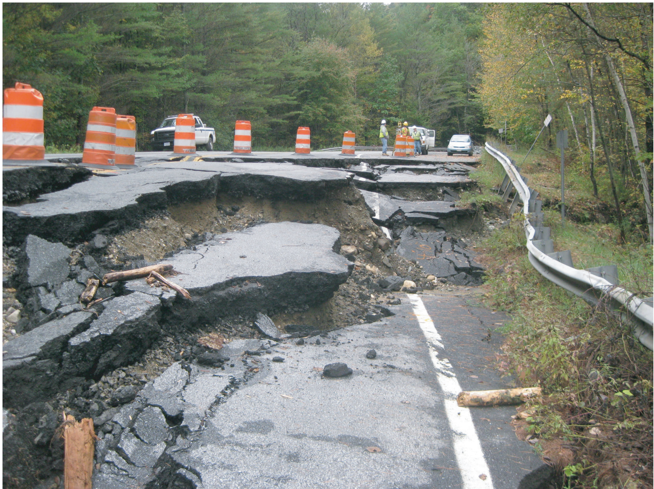
Rotational slide at site 1. Road built on lake-bottom sediments overlain by debris flow and alluvial deposits from Trout Brook. Area has had chronic failures due to erosion of toe of slope by the Cold River during periodic flooding, high pore pressures, poor strength soils and added weight due to heavy rains. Area affected is about 800 feet.
