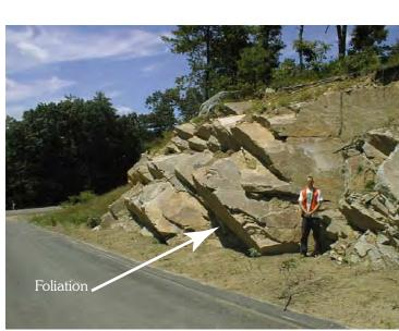
**Example of Steeply-Dipping Layered Rocks** Foliated binary Andover granite showing three well-developed fracture sets. Partings parallel to foliation are strongly developed. Rock breaks into characteristic rhombohedral blocks.
