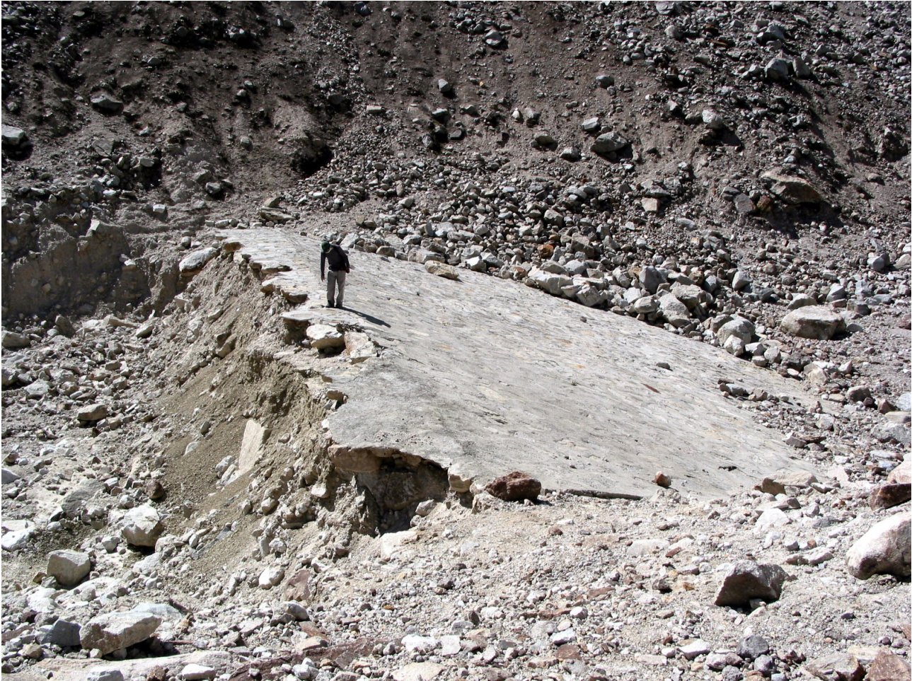
Figure 4. Lake Palcacocha security dam in 2003 that was partially destroyed when a landslide fell into the lake and created waves that overtopped the dam. Photo: M. Carey.
